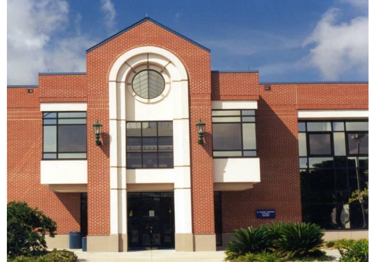
W. Richard Johnston Technical Building Entry Red Brick & Painted Stucco
