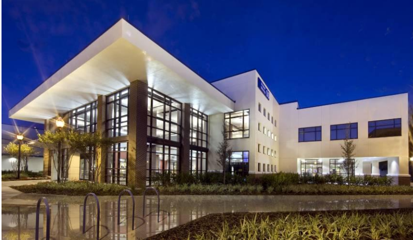
Student Services Building Brick Details & Painted Stucco
