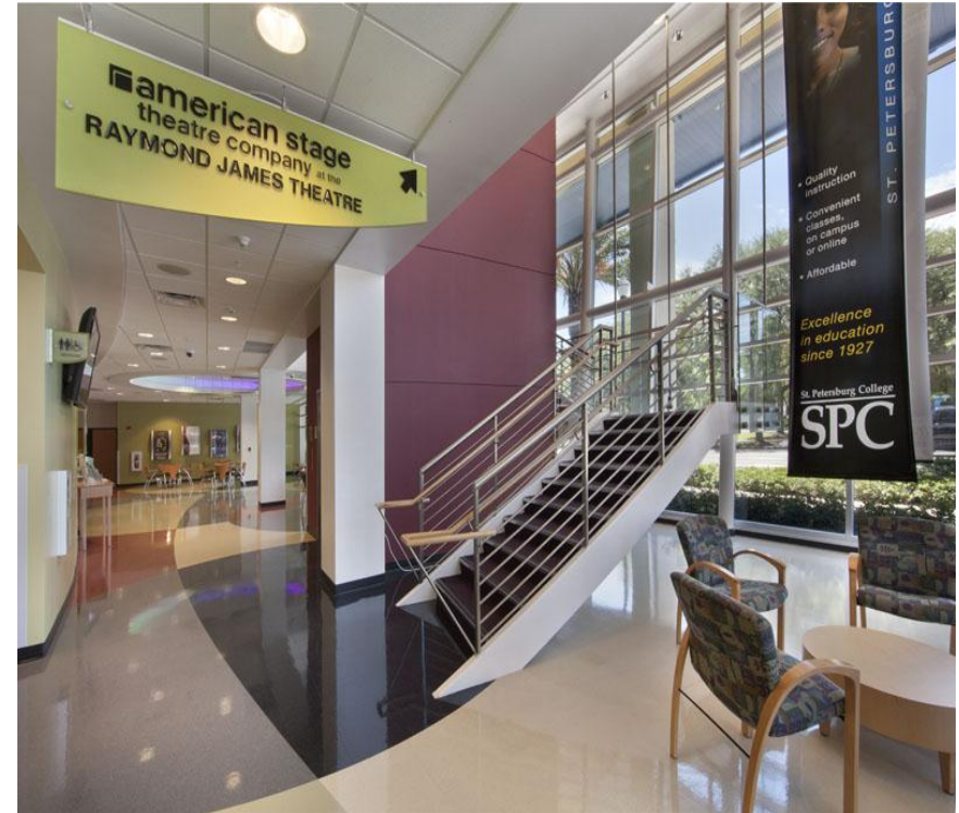
Stainless Steel Guardrail w/ Hardwood Handrail Eco-Resin Signage
